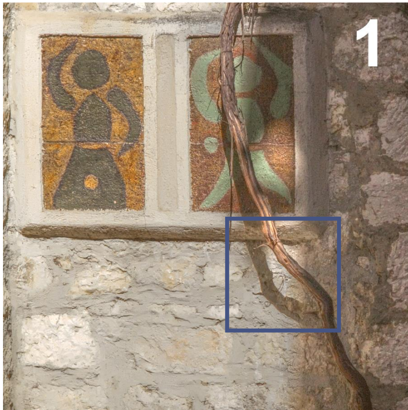
Progress of restoration
